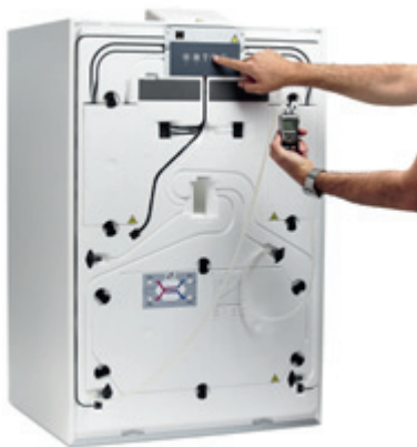
CALIBRATION USING CONTROL PANEL
